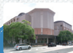
Nagasaki Brick Hall
